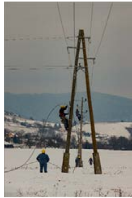
Hanging optical cable in the direction towards Bizeljско Author: Davor Lipej
